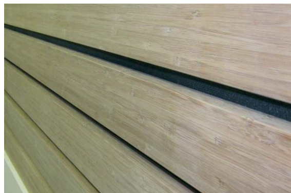
BCL bamboo cladding panel in-situ
